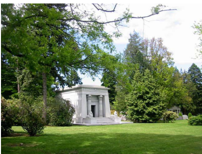
Egyptian Revival mausoleum architecture at Woodlawn
